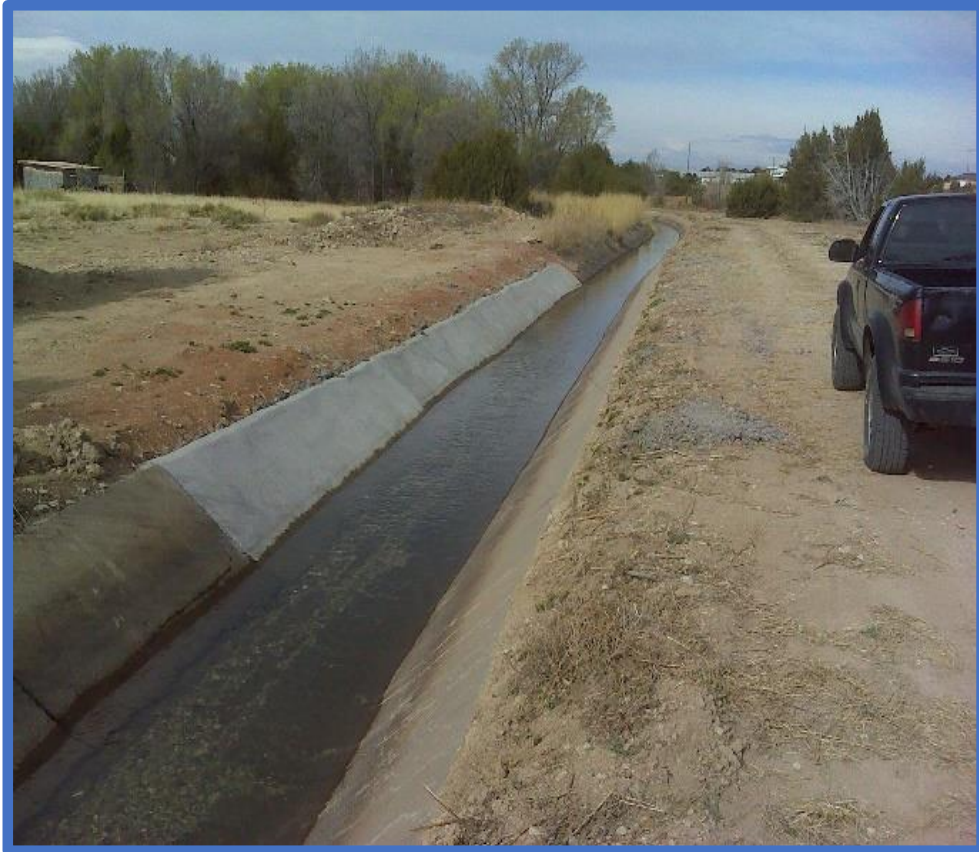
Beaver Park Upper Canal – New canal concrete lining sections functioning. April 2018.
